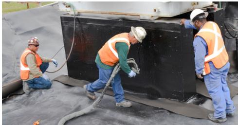
Sealing transformer pad with PolySeam.
