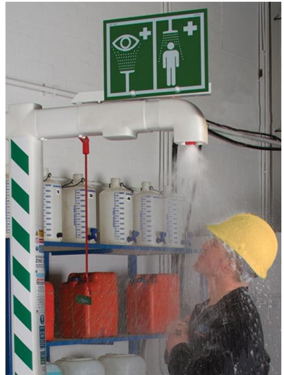
Heated and insulated for frost protection.
